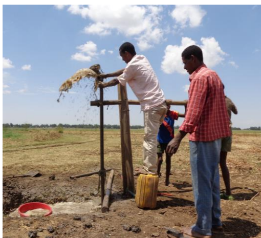
Figure 1 Manual drilling using simple sludging method - Fogera floodplain Ethiopia (source MetaMeta)
