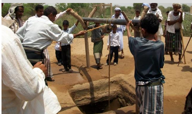
Figure 2 Hand dug-well in equipped with lifting mechanism, Yemen (source Oxfam UK).
